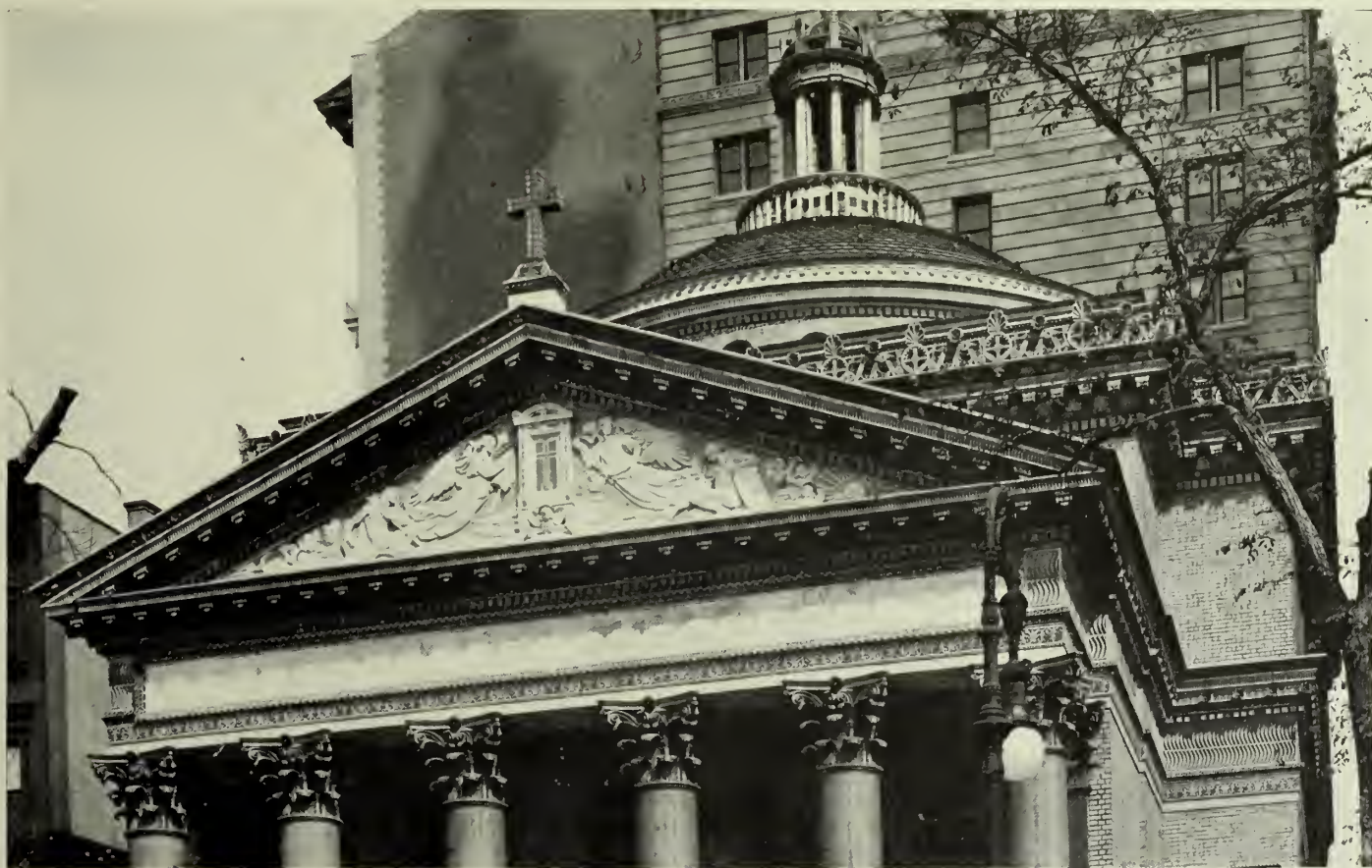
PEDIMENT OF MADISON SQUARE PRESBYTERIAN CHURCH, NEW YORK CITY. Showing new panel executed in polychrome terra cotta by the Atlantic Terra Cotta Company.
